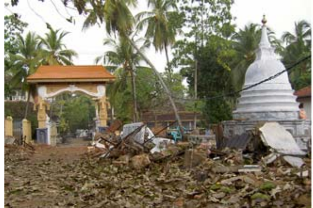
A Buddhist Temple in Galle, Sri Lanka stands in the midst of the tsunami rubble
